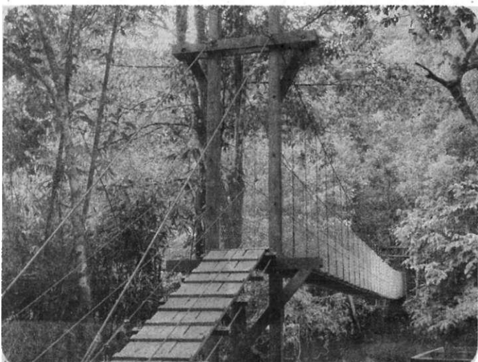
The completed suspension bridge at Ba' Medamot
