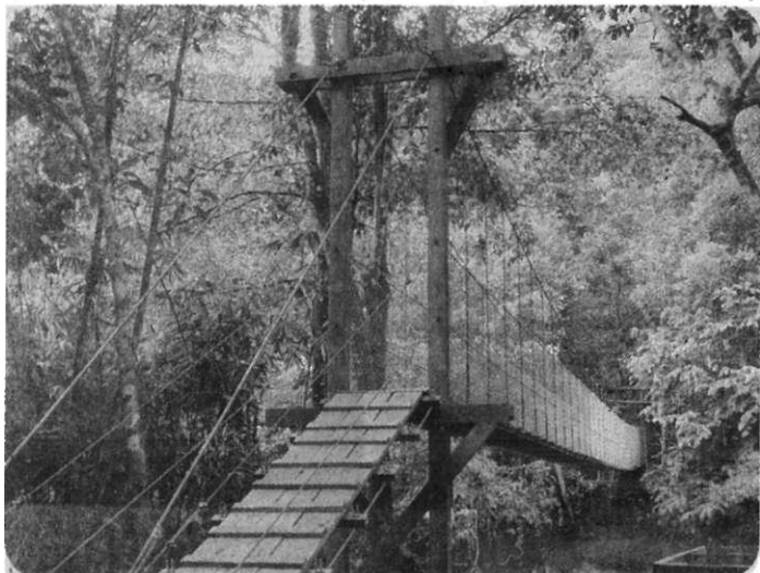
The completed suspension bridge at Ba' Medamot
